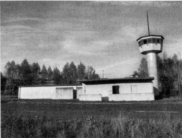
Support area watch tower.
